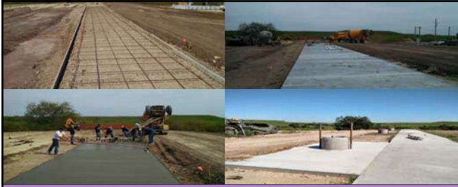
Pouring Concrete Culverts, setting posts
